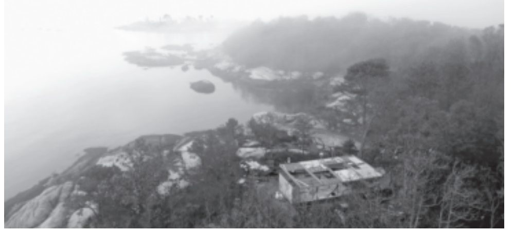
Building Lab, Horse Island Coastal Research Station under construction, Connecticut, 2021
