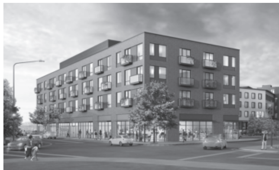
Newman Architects, project of Melinda Agron, rendering of 500 Blake Street mixed-use development, Westville, New Haven
