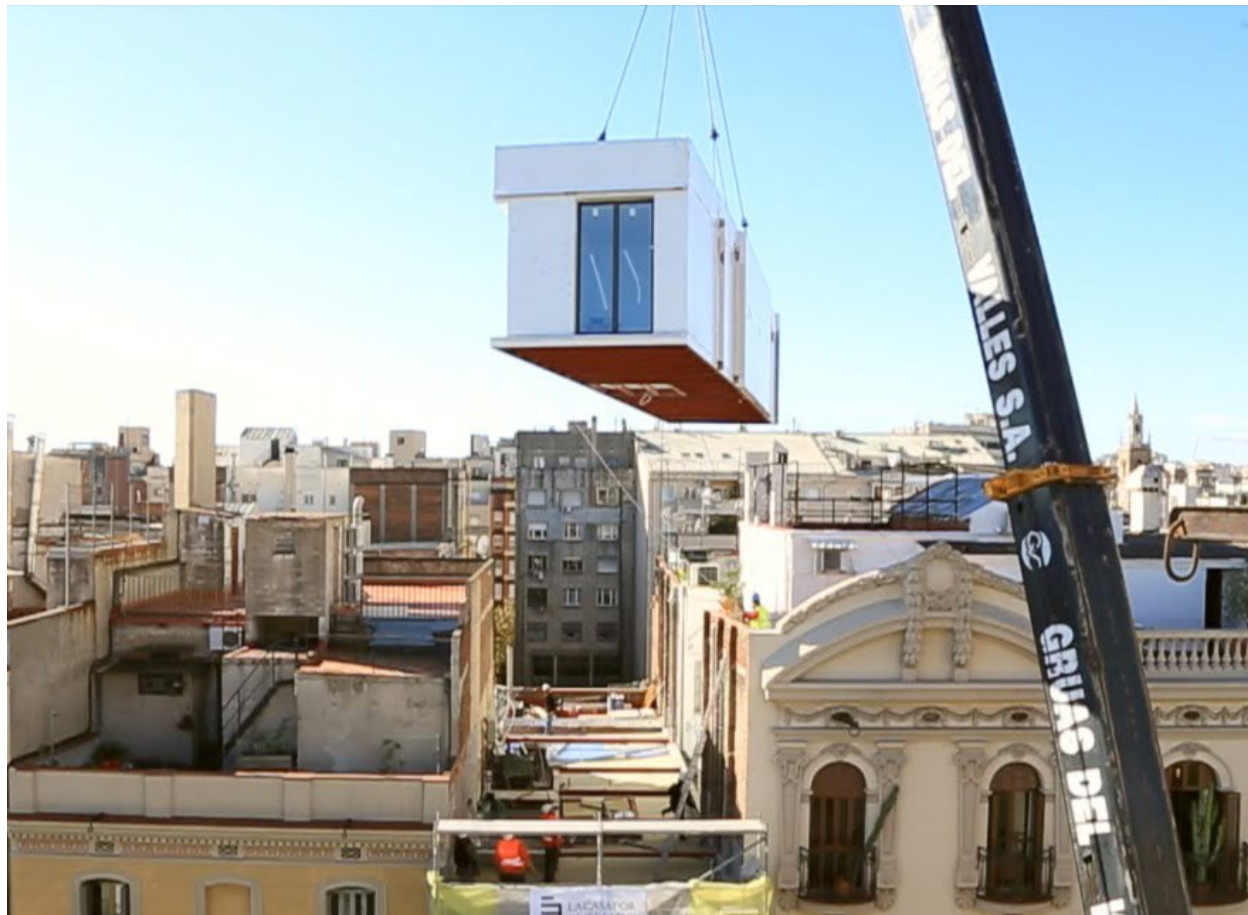
Image 6 | La Casa por el Tejado, rooftop ADU project in Barcelona. Modular rooftop unit being lifted into place by crane.
