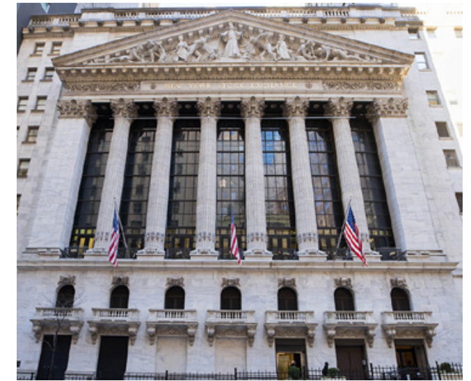
Figure 1. New York Stock Exchange Facade. Photo credit: nyse.com
