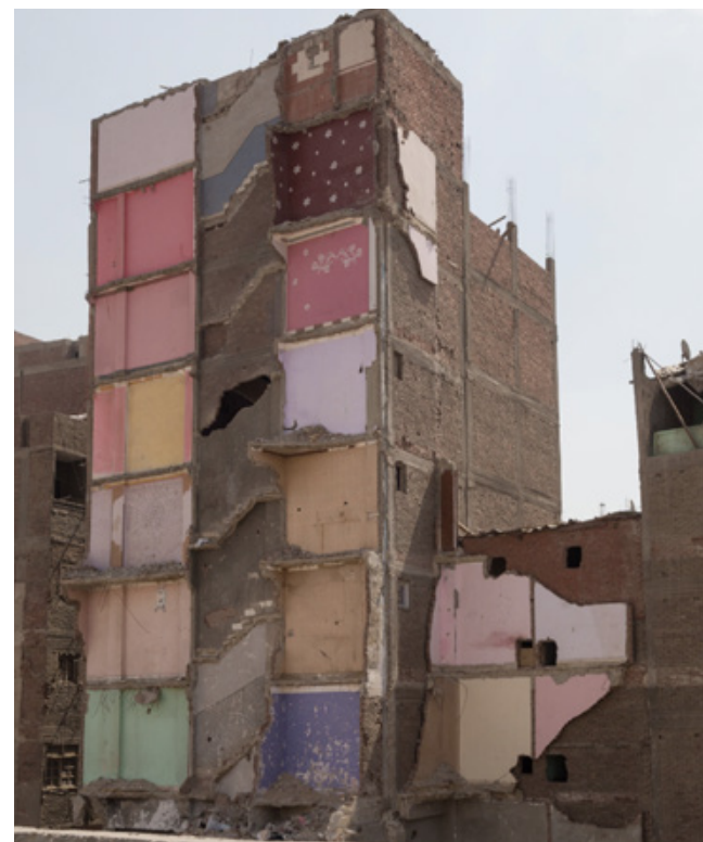
Figure 4. Building undergoing demolition. Photo credit: Yasmine El Rashidi
