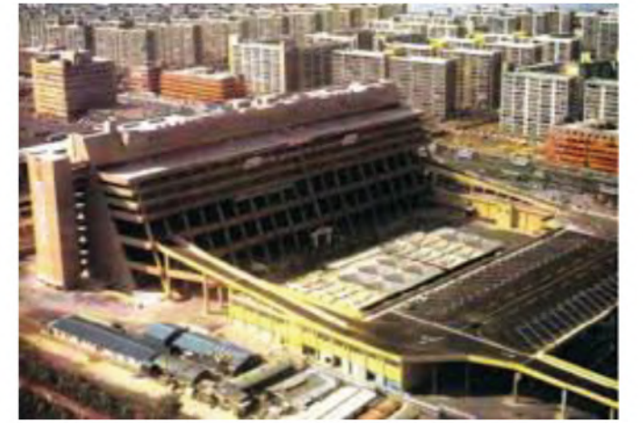
The Express Bus Terminal is part of Seoul's patrimony; an 80's brutalist building with a unique sloping facade and ground level colonnade. Working with these elements, the proposed geometry is intended to be a powerful strategy for combining elements in the site. At the central axis of the project area, a split uncovered area brings light to the underground.
