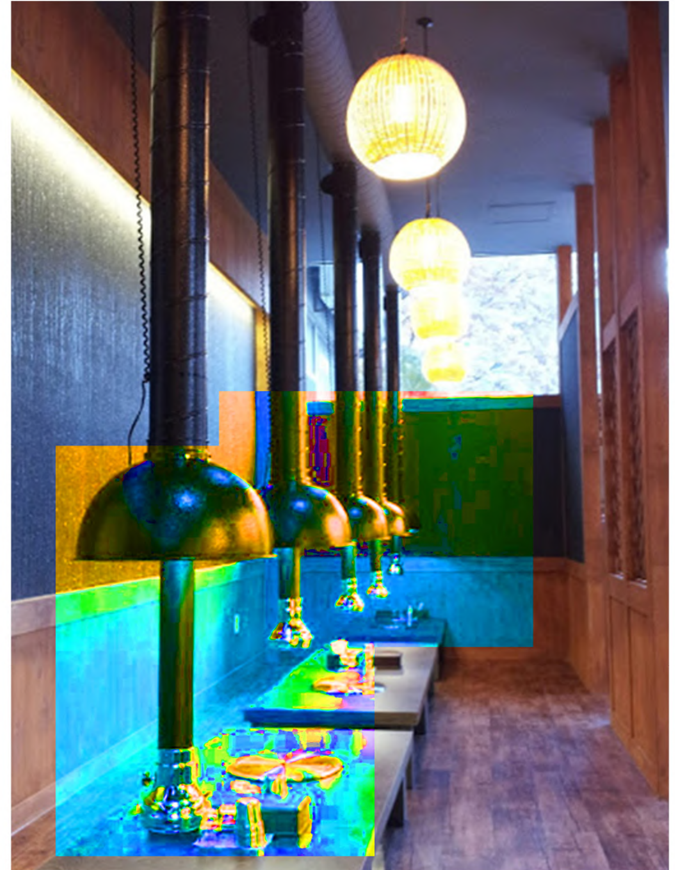
The idea was inspired by individual ventilation system in Korean BBQ restaurant. This is a facility that is placed in a local area and changed in a flexible manner, rather than a system that circulates large spaces at once.
