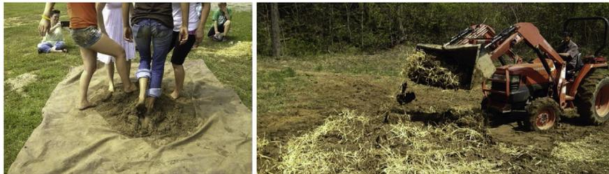
Fig. 2. Manual cob production (left) and tractor-cob (right) [9].
