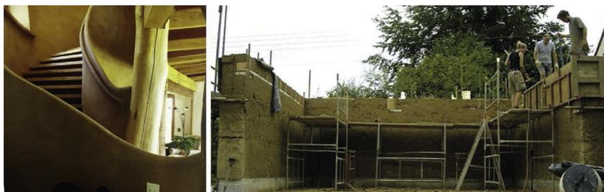
Fig. 3. Sculptural cob wall (left) and shuttered-cob (right) [9,16].
