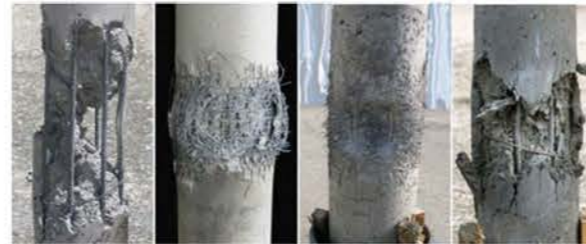
Columns after detonation experiment (reinforced concrete, DUCON, SIFCON, UHPFRCC) [13]
