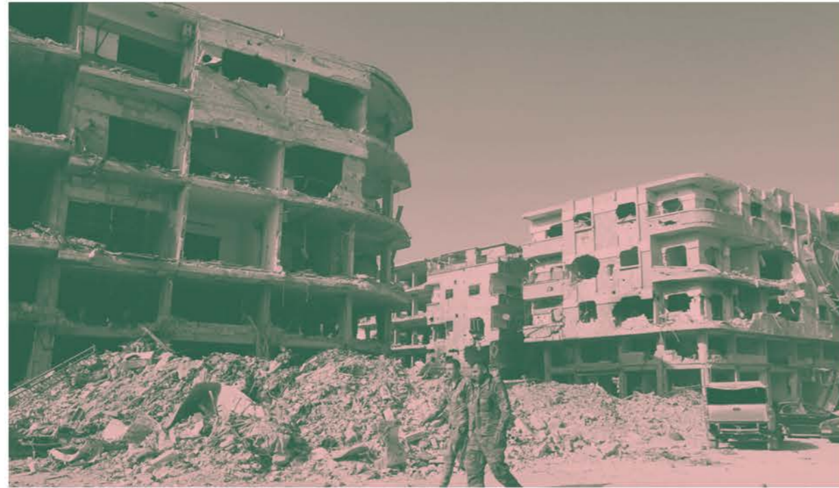
“Syrian government forces on a destroyed street in the Hajar al-Aswad area on the southern outskirts of Damascus” [10]
