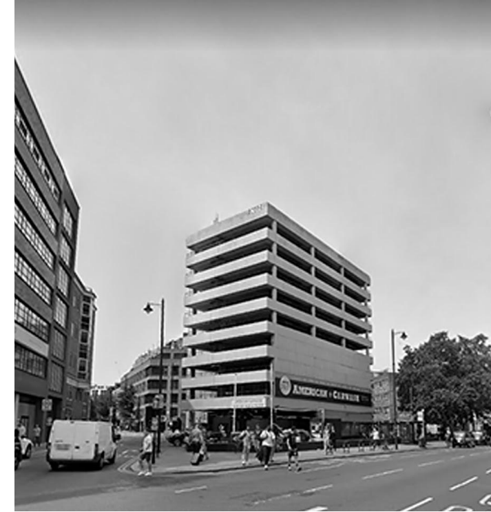
the existing building
