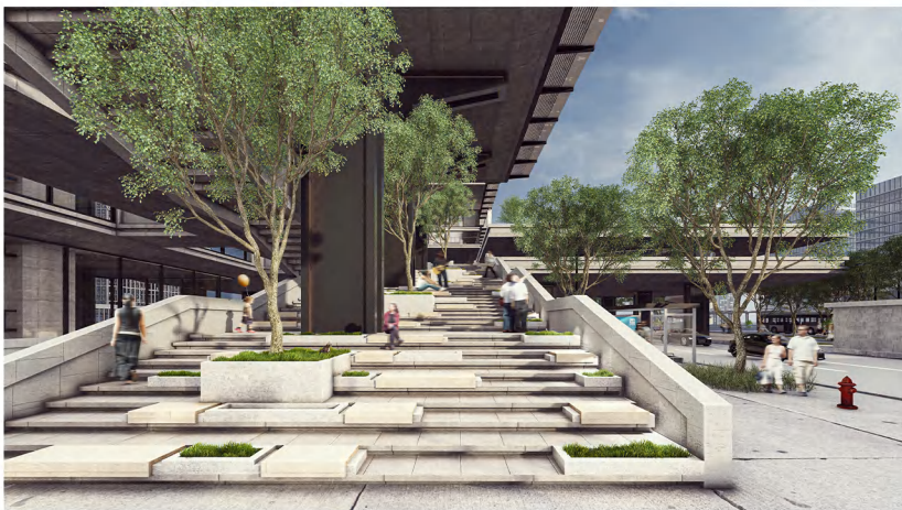
This is a large landscape step. Since the original columns were very dense, we removed several original columns to keep the space open and reinforced the retained columns.
