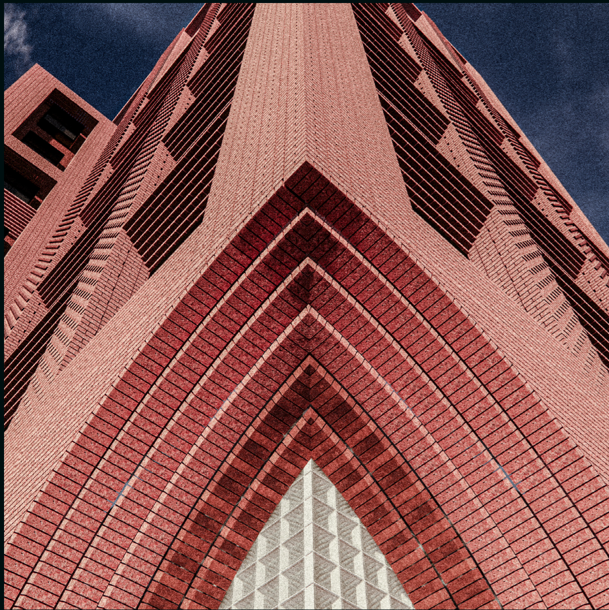
Contrast between the existing brick arrangement and new brick typology.
